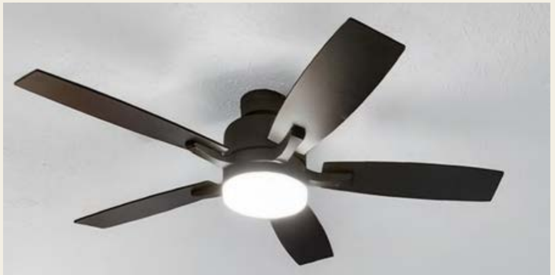
Black 5 Blade Ceiling Fan Installed
