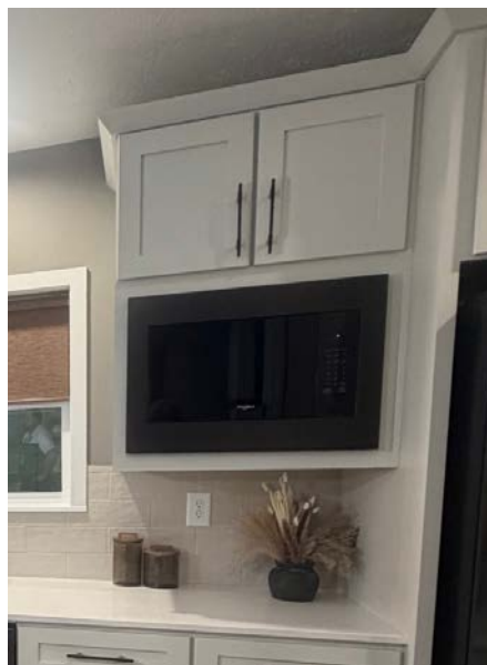
Built-In Microwave in Overhead Cabinet
