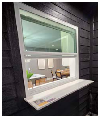
4034 Porch Service Window
