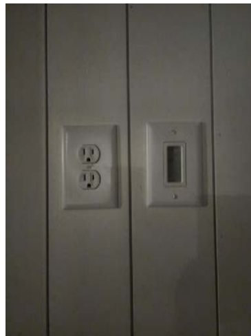
Cable Access Wall Plate 1-high & 1-low
