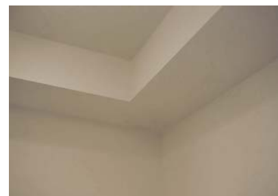
Drywall Tray Ceiling - Where Available Ceiling Cove N/A
