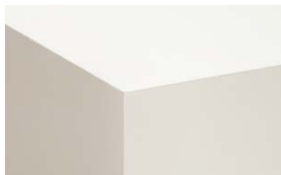
Finished Ceiling Joint
